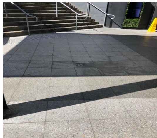
Figure 6. Non-compliant Cross falls
